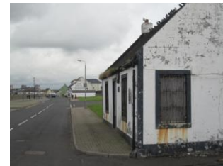
Fig.9-17 Harbour Master's House, in background, Ship Inn, 2013
