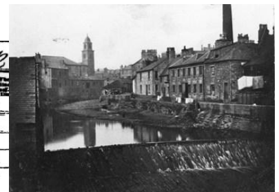
Fig.6-4 Kilmarnock Water, Sandbed St & Nelson St, & Laigh Kirk
