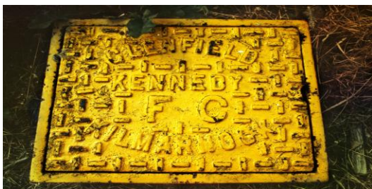
Fig.6-16 Glenfield Kennedy Fire Hydrant Cover.
