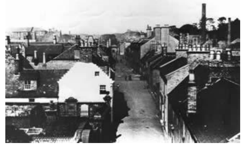
Fig.6-6 High Street, Kilmarnock.
